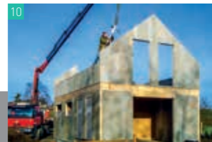
10 Assembly of PURLIVE bearing structures
