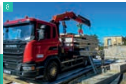
8 Delivery of building elements to the construction site
