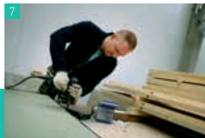
7 Fabrication of PURLIVE building elements
