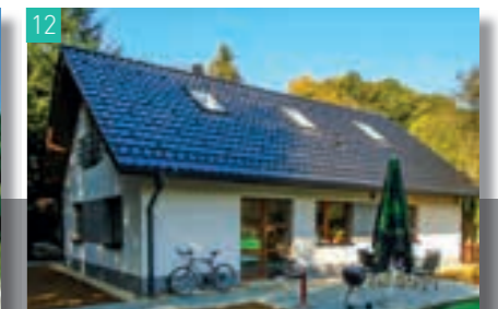
12 Completing a key-turn construction
